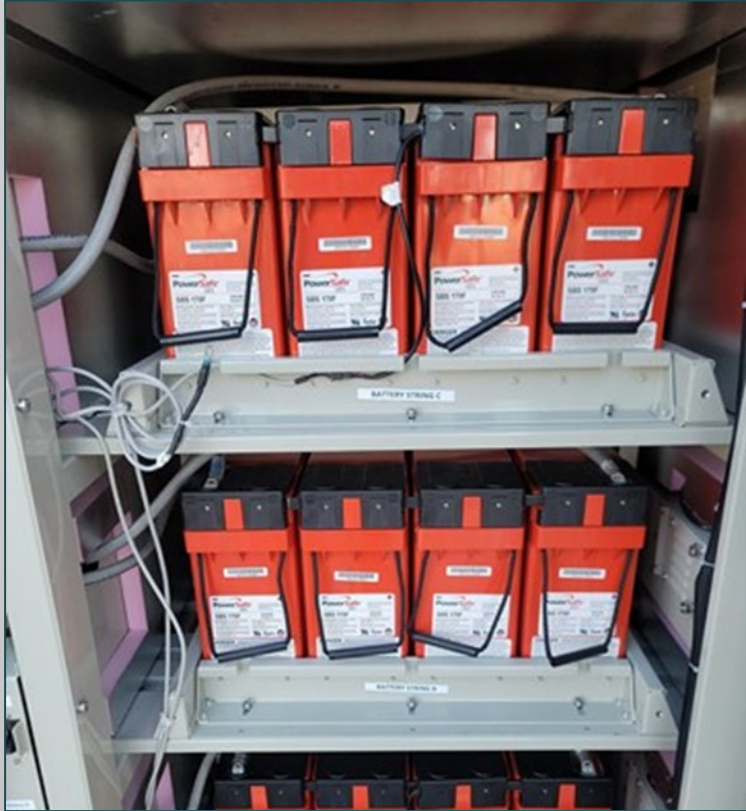
24 VDC Batteries
